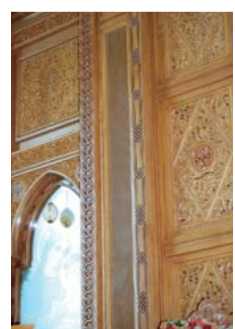
A Messenger XL array concealed within the main church
